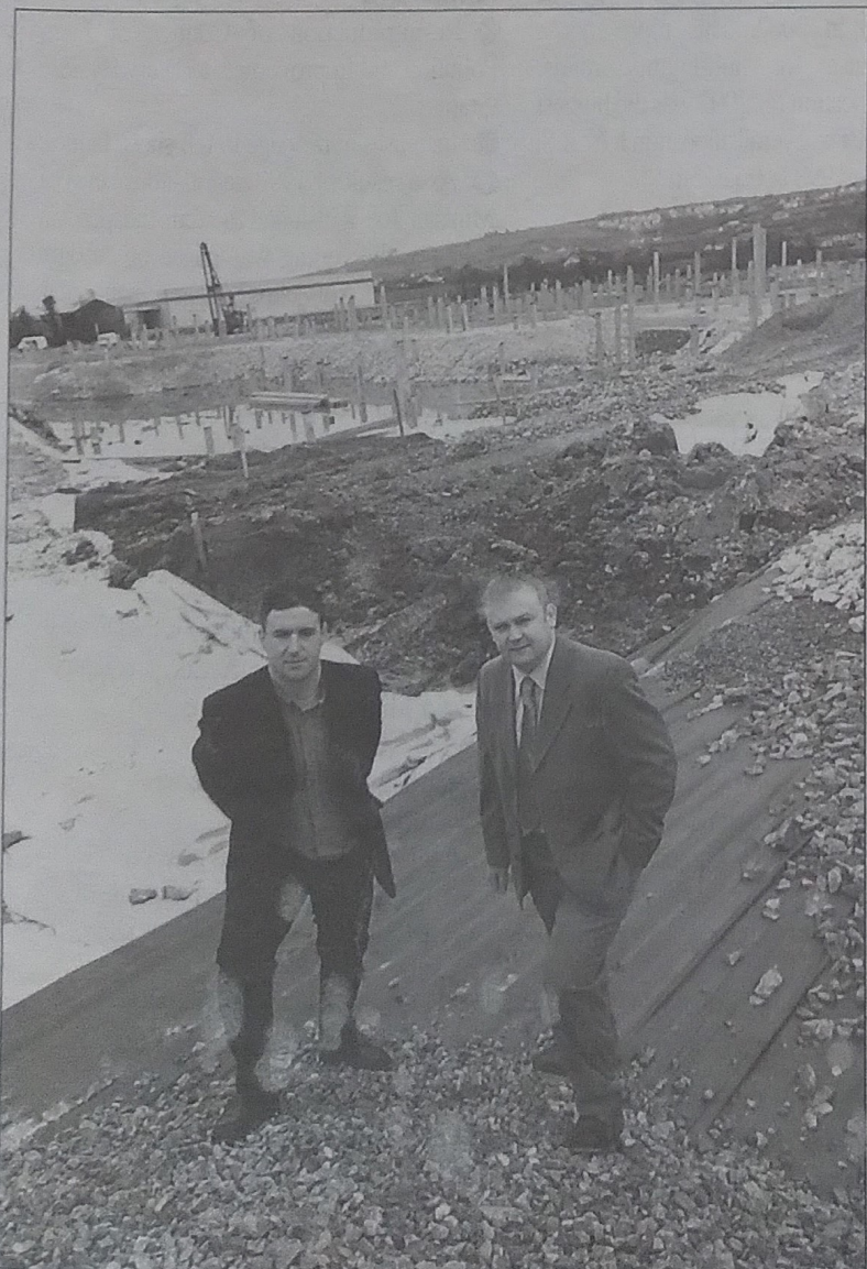
Cllr. Niall Blaney and Cllr. Dessie Larkin at the site of the new Letterkenny Sports Complex.
